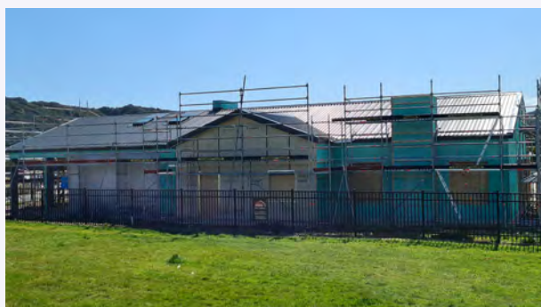
Wainuiomata Hub under construction
