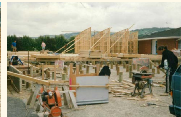
Constructing framework for the addition bedrooms of the John Muir wing
