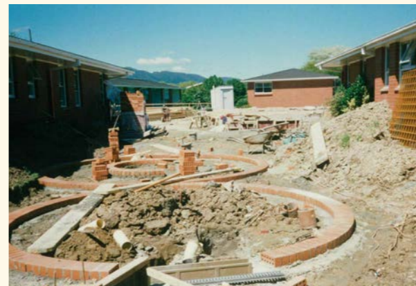
Work underway to complete the courtyard near the John Muir wing
